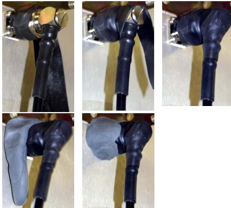
Figure 15 Waterproofing Outdoors Connections
