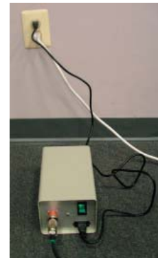
Figure 1-13. Placement of Transformer
