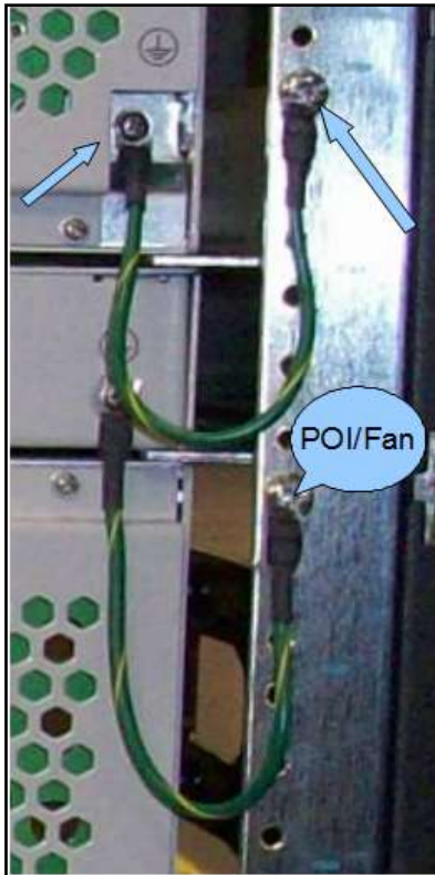
Figure 4-21. Grounded Host Unit (shown with optional POI Unit, also grounded)
