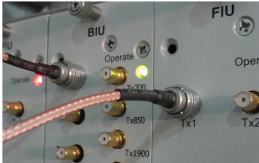
Figure 24 BTS QMA Coaxial Cable Connection
