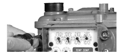
Completely remove and discard the old gasket. Use a putty knife to clean the meter surface of all gasket remnants that might limit the effectiveness of the new gasket.
