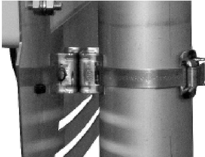
Figure 7: Close up of right side Band-IT connection
