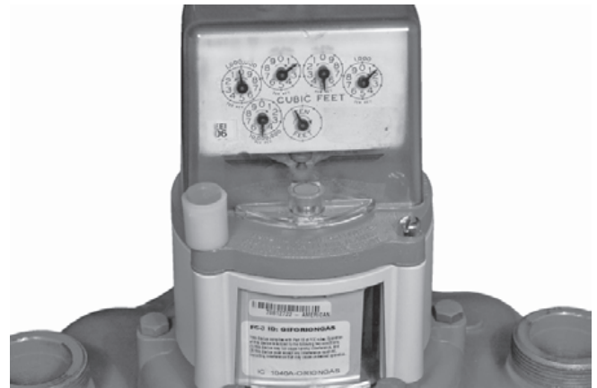
After Installation of ORION Transmitter
