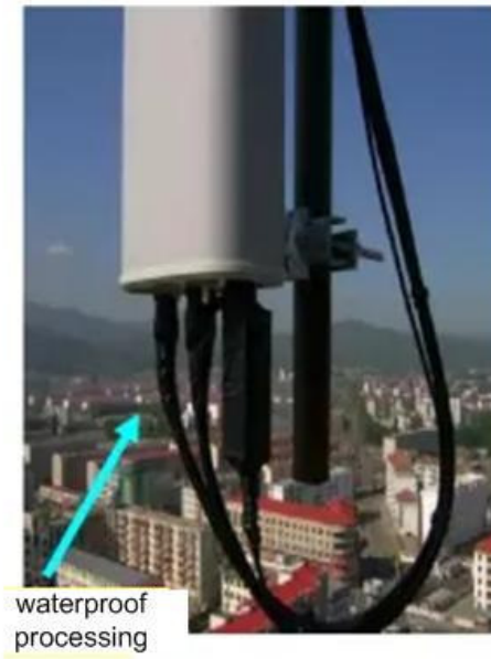
Figure 3-13 Antenna Waterproof Protection
