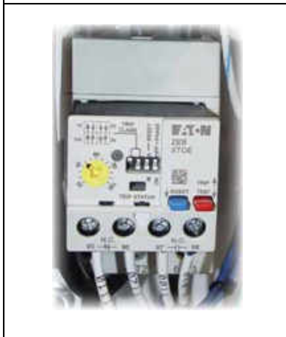
Figure 6-7 Overload Relay (typical)
