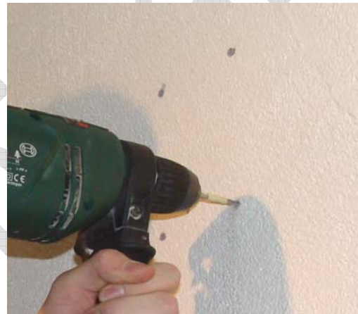
Figure 4-2: Drilling holes
