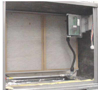
Fig. 25 - Return Air Sensor Operating Position
