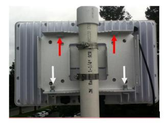
The installer can attach a rope or hook to one of the holes on the side of the mounting bracket in order to hang IBR on a utility belt until it is time to attach it to the bracket. To aid in hanging IBR, the plate on IBR can be hooked onto the mating wall/pole plate while the two M6x10 mounting bolts are being tightened. An Allen wrench is needed to tighten the bolts.
