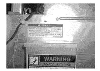
**FIGURE 47:** Install danger label on vestibule panel just below upper limit switch.
