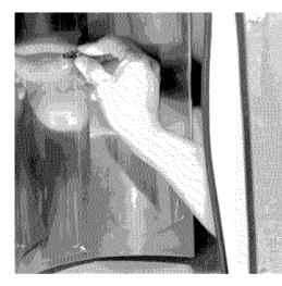
**FIGURE 21:** Install stainless steel nuts found in hardware bag. Do not tighten.
