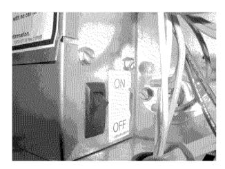
FIGURE 2: Turn power switch to off position.
