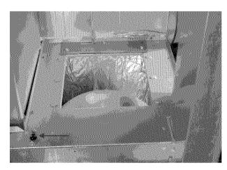
FIGURE 33: Remove wires from upper limit.
