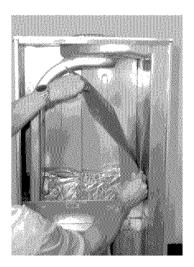
**FIGURE 36:** To protect side wall insulation insert cardboard sheet as a "shoe horn" to insert auxiliary limit switch assembly between insulation and heat exchanger.
