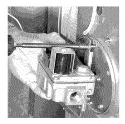
FIGURE 29: Reinstall gas valve and gas piping.
