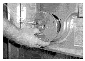
FIGURE 4: Burner assembly removal
