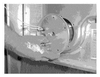
FIGURE 28: Reinstall burner.
