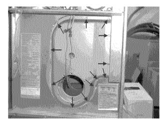
**FIGURE 26:** Install burner inlet pan with 12 screws. If needed, re-seal pan with high temperature RTV silicone.
