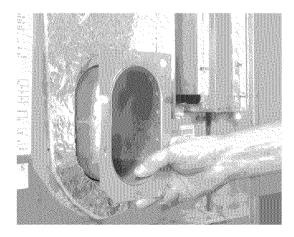
FIGURE 24: Reinstall burner chute to original position.
