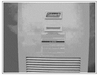
**FIGURE 50:** Install Consumer Notice on top front furnace door and instruct the consumer on how to properly maintain their furnace.
