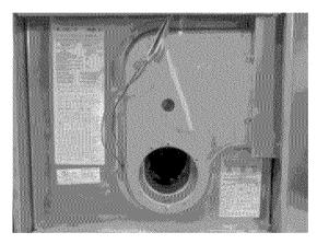
FIGURE 11: Remove pressure switch tube.
