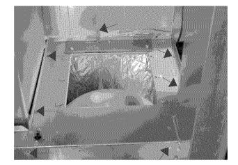
FIGURE 34: Remove blower support shelf (7 screws).
