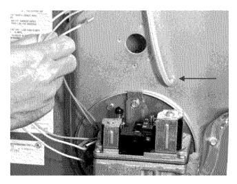
**FIGURE 30:** Reconnect pressure tube to pressure switch and wiring connectors to gas valve, igniter and sensor.
