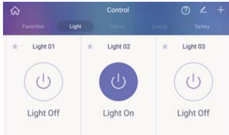
[Lighting Control Screen]
