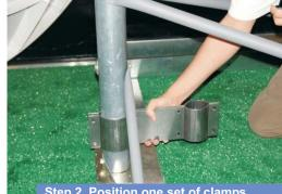
Step 2. Position one set of clamps around the center satellite pole. Partially screw in eight of the bolts. Leave space to slide in the adjacent pole.
