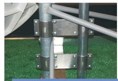
Step 3. Slide the adjacent pole between the clamps. Fasten the bolts. Position the second set of clamps around both poles and fasten the remaining bolts.
