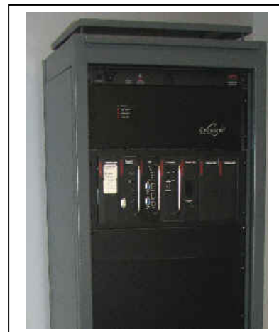
Figure 2 - Typical rackmount installation of radio modem and Crescent PA
