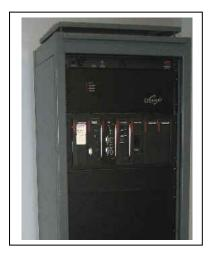
Figure 2 - Typical rackmount installation of radio modem and Crescend PA
