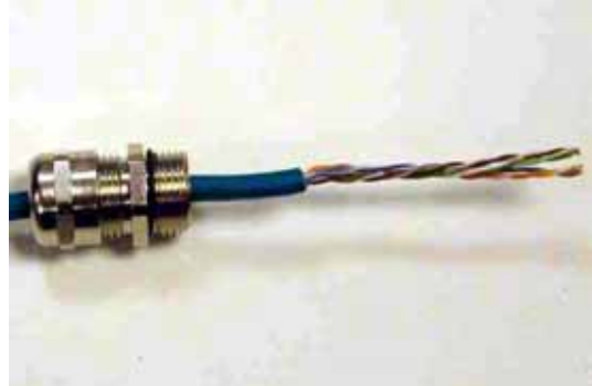
Step 2: Strip the outer insulation
