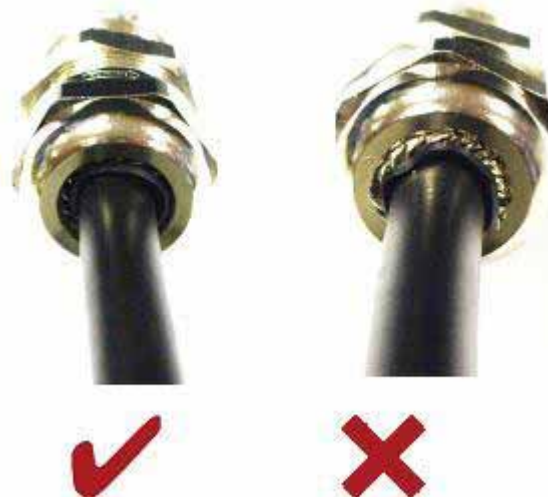
Figure 43 - Correct and Incorrect Tightening of Cable Gland
