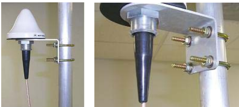
Figure 43 GPS antenna mounting
