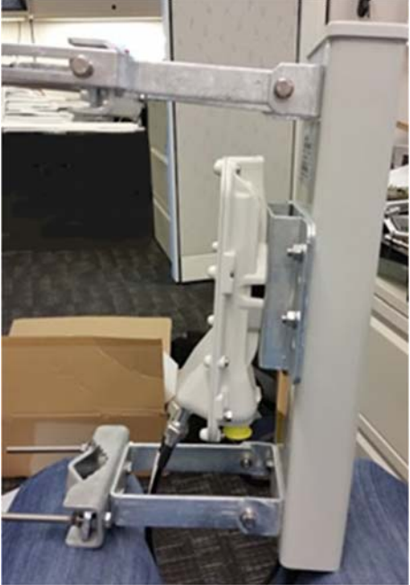
Figure 88 Completed AP and antenna assembly
