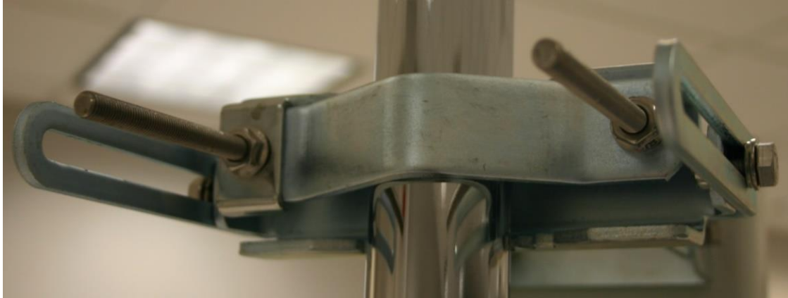
Figure 78 Attaching the AP antenna upper bracket to the pole
