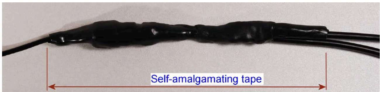
Figure 100 Wrapping self-amalgamating tape around the GPS adapter cable joint
