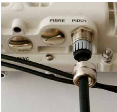
Step 3: Screw in the body of the weather proofing gland and tighten
