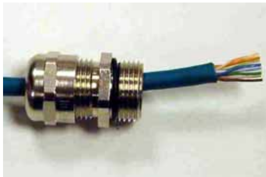
Step 3: Arrange conductors as shown in fig. A2 and cut to length
