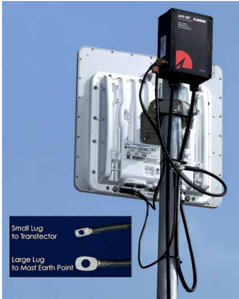
Figure 110 - Upper Grounding Configuration
