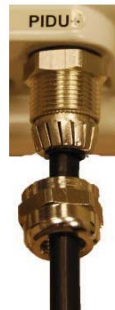
Step 3: Screw in the body of the weather proofing gland and tighten
