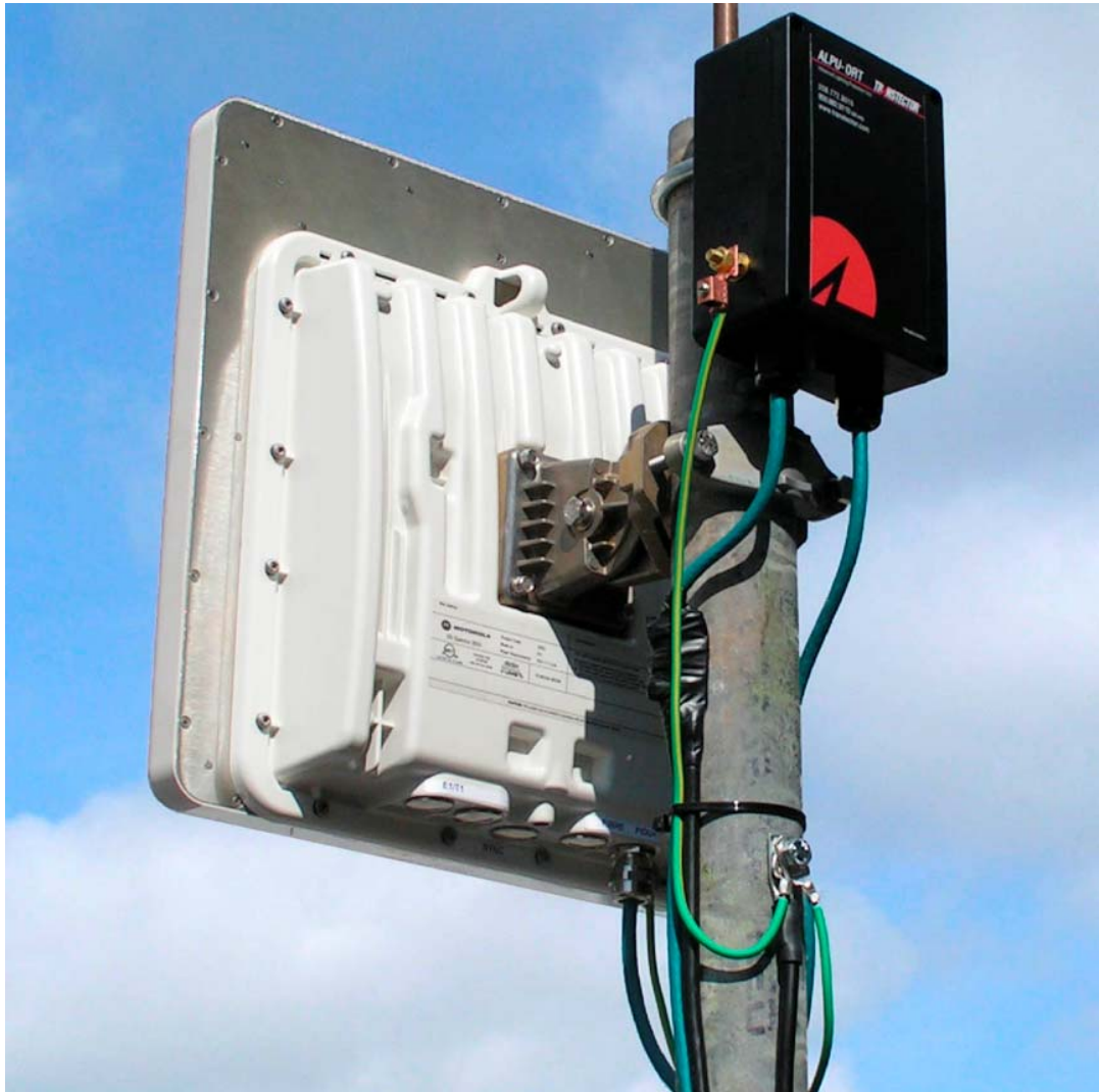
Figure 79 - Upper Grounding Configuration
