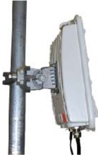
Figure 21 - ODU Mounted on Pole
