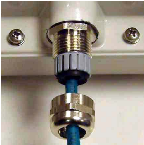
Step 3: Screw in the body of the weather proofing gland and tighten
