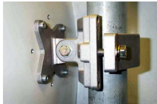
Step 2: Mate the unit to the bracket together and tighten the nut and bolt.
