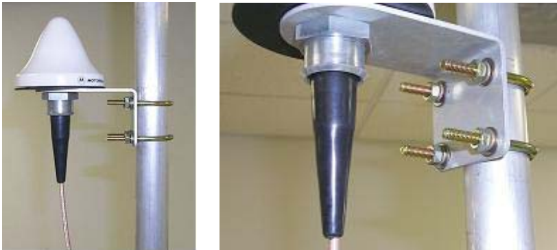
Figure 29 GPS antenna mounting
