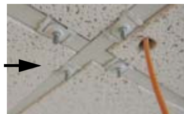
T-Bar Clips (4 shown; only 2 needed)
