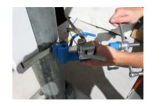
Using the built in cutting tool on the Band-It tool, cut the excess strap.
