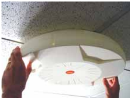
Figure 44. Attaching the Unit (XS-3900)
