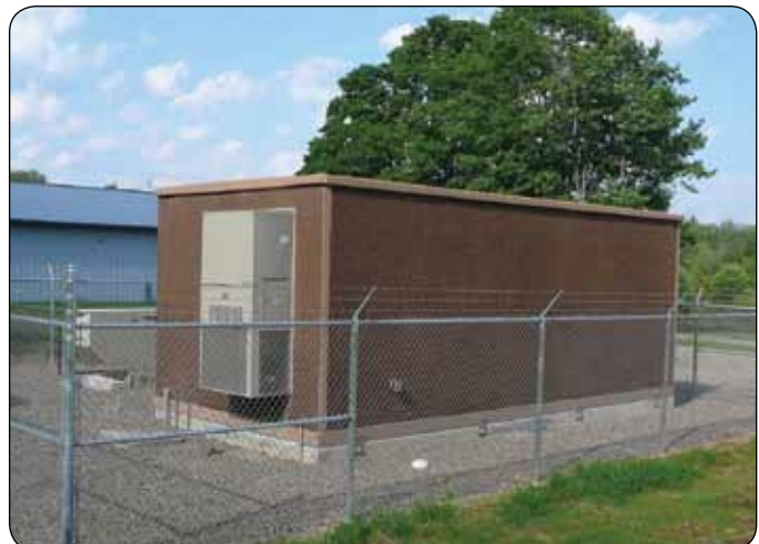
Site completion including landscaping, fencing and security.
