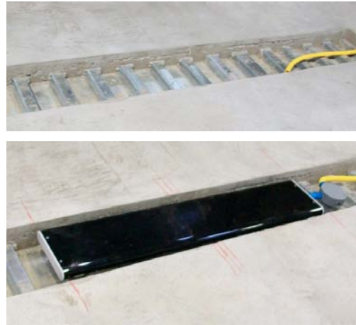
Figure 3.4 Antenna Installed (not buried until after testing)
