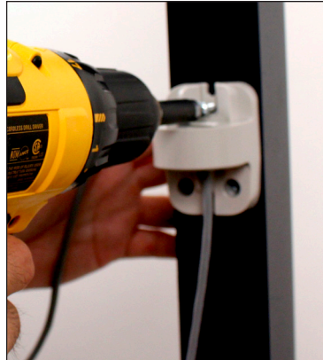
Figure 2 - Screw in bottom Bracket.
