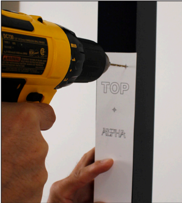
Figure 1 - Drill holes as indicated on template.
