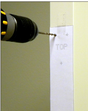
Figure 1 - Drill holes as indicated on template
