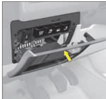
Access to the first fusebox under the dashboard
