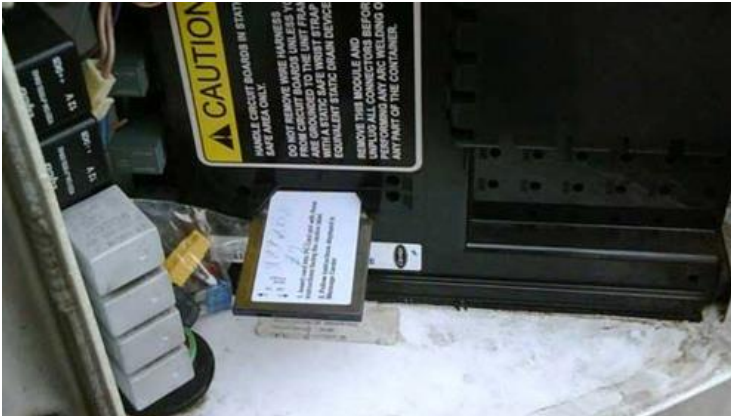
Picture 11: Carrier Datacard in Controller PCMCIA Slot
