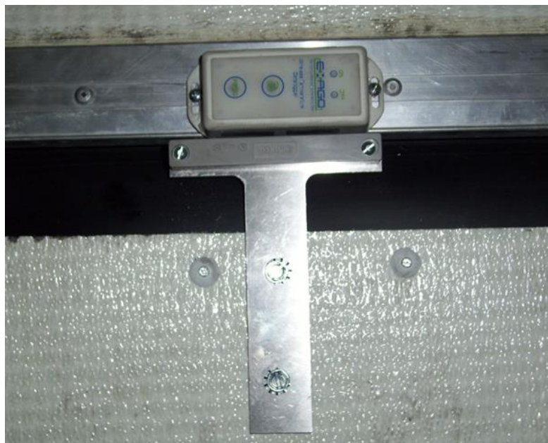
Door Tag and Magnet fitted to Barn or Side Door
