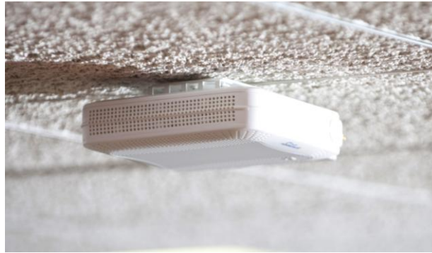
Figure 5-2. VAP Installed Horizontally on Ceiling
