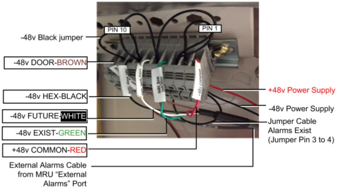
Figure 4-13. Example of External Alarm Wiring Connections
