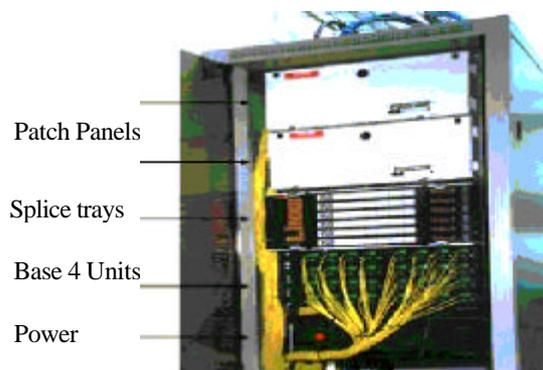
3. Near Modular Base Unit, install patch panel cabinet (**SC/APC** adaptors) for fiber optic cable connections.
