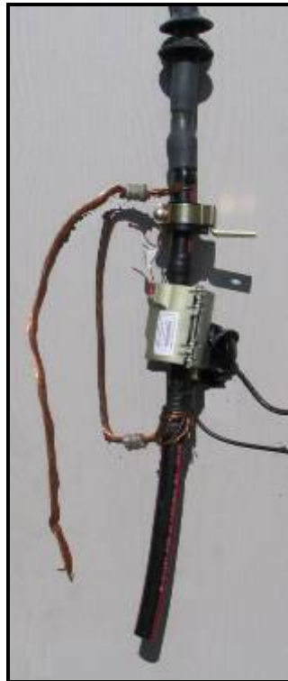
Figure 28 – CT Coupler URD 5010rp installed
