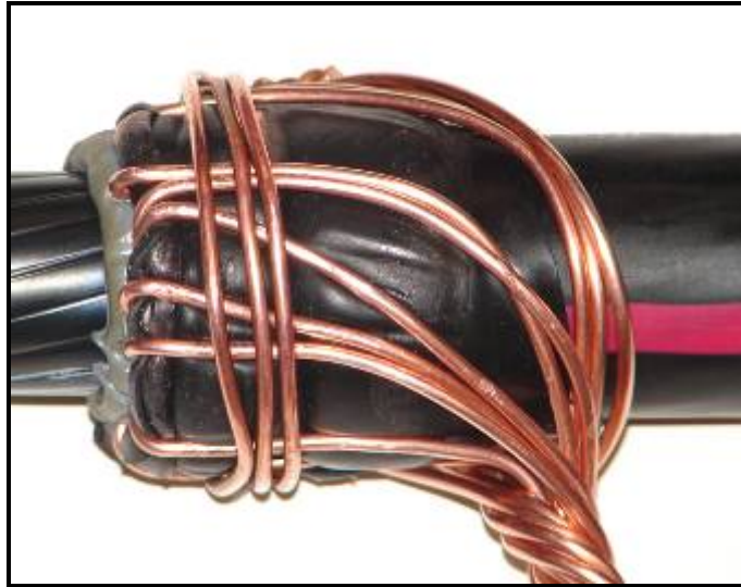
Figure 23 – Neutral Wires wrapped concentrically
