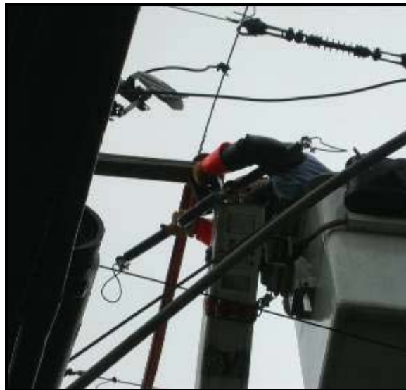
Figure 16 – Attaching CT Coupler to Cross Arm
