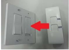
Step 3, secure the ZSC tightly by pressing firmly on the existing wall plate
