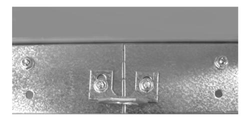
9. Use the drawing below to cut the hole in the duct. Fasten the module to the edges using screws.
