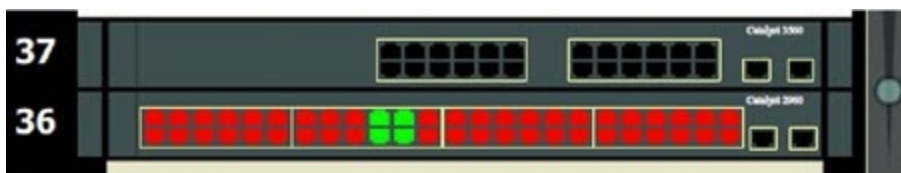
Figure 222: Deployed switch showing red and green port status icons
