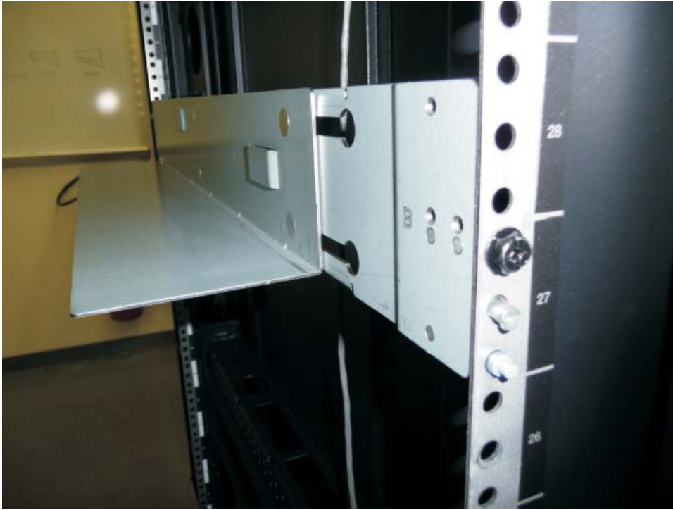
Figure 4-10. Rear view of Rack Kit B shows a different mounting method
