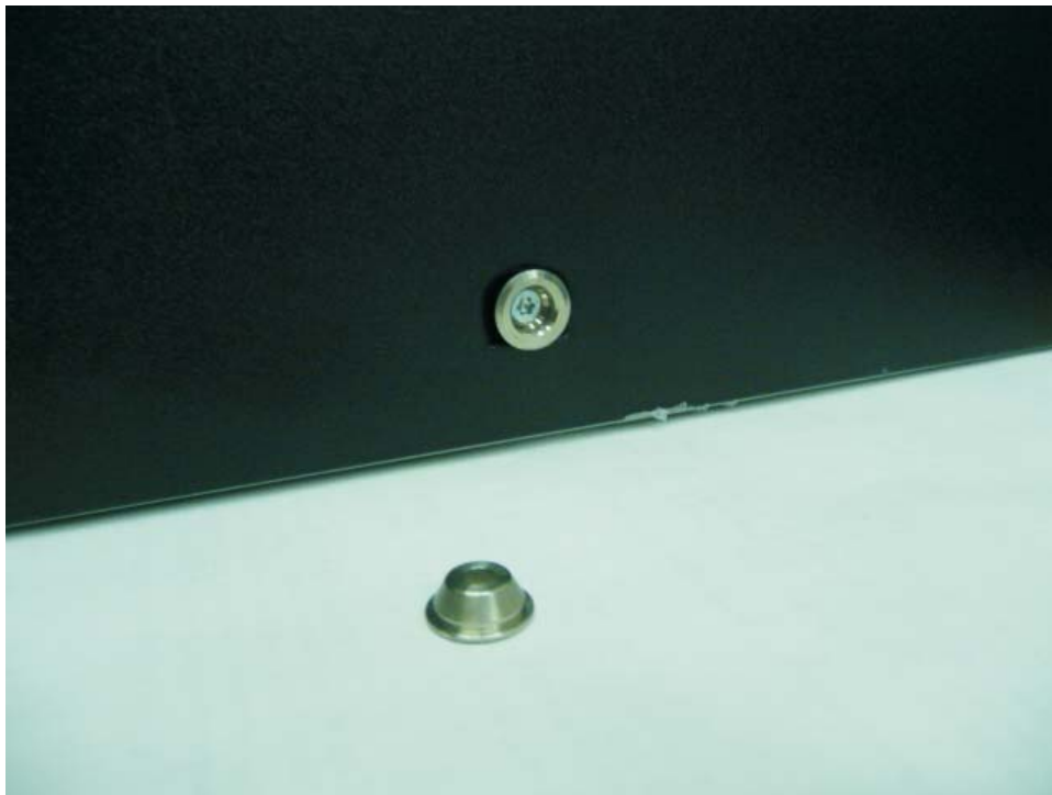
Figure 4-13. Close-up view of mounting of the anchors on both sides of the library
