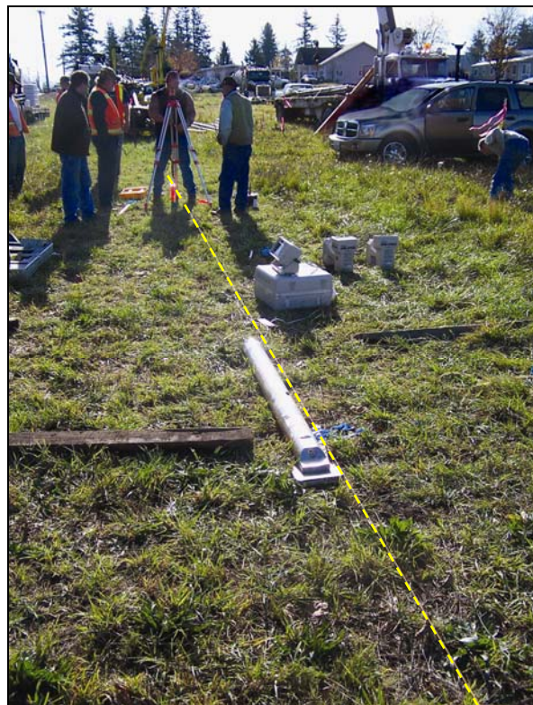
Aligning Drill to Marked Borepath
