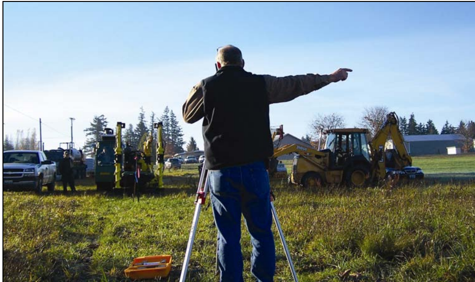
Aligning Drill to Marked Borepath
