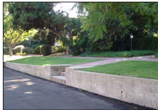
Figure 2.39: Seventh Avenue retaining wall at roadbed, Hillcrest, Crittenden's Addition.
