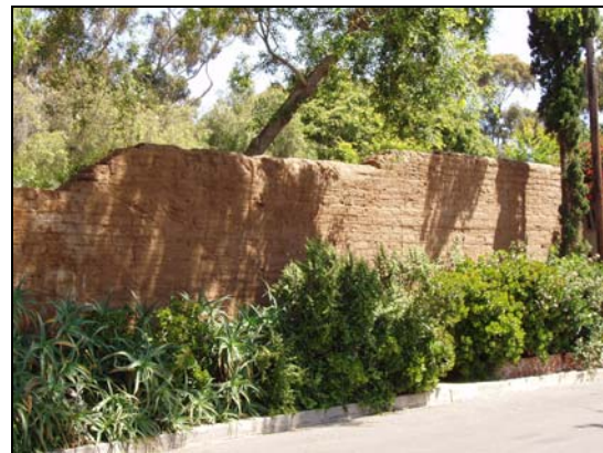
Figure 2.5: Pioneer Park & WPA Adobe Wall.
