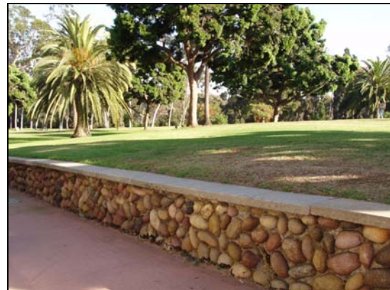
Figure 2.40: Balboa Park Cobble Wall, Upas St./Sixth Avenue, Hillcrest.
