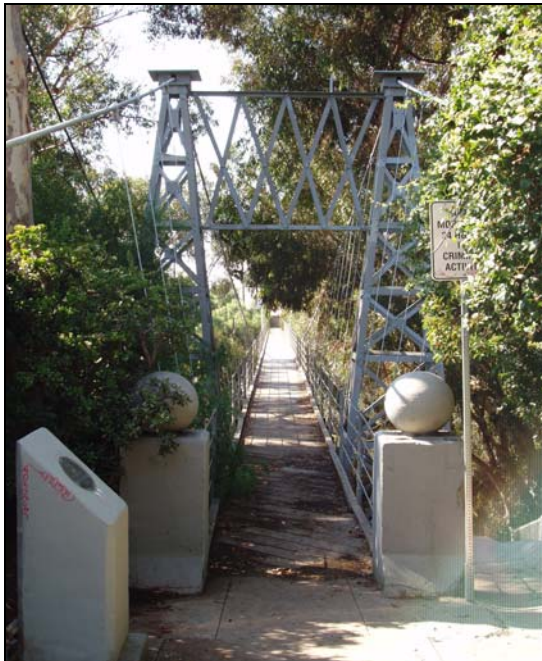
Figure 2.23: Spruce Street Suspension Bridge, 1977.
