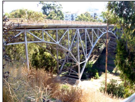
Figure 2.25: First Avenue Bridge, 1993.
