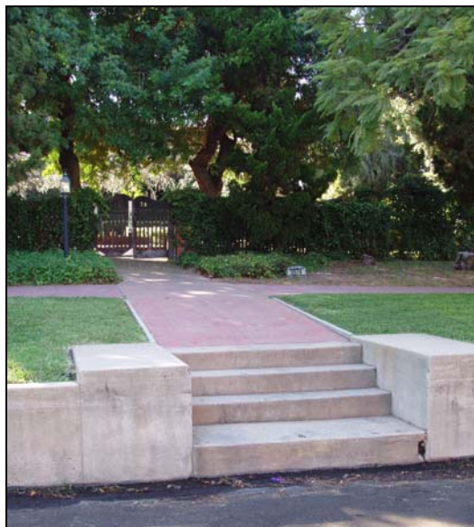
Figure 2.19: Retaining Wall/Stairs at Street.
