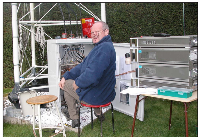
Fig 9-77 —The base of ON4UN’s 160-meter vertical and the cabinet housing both the 80-hybrid-coupler Comtek and WX0B Lahlum networks for the 80-meter Four Square. R. Vermet, ON6WU, with his professional antenna measuring setup, tunes the 80-meter vertical. An HP network analyzer is used that directly produces a Smith Chart.
