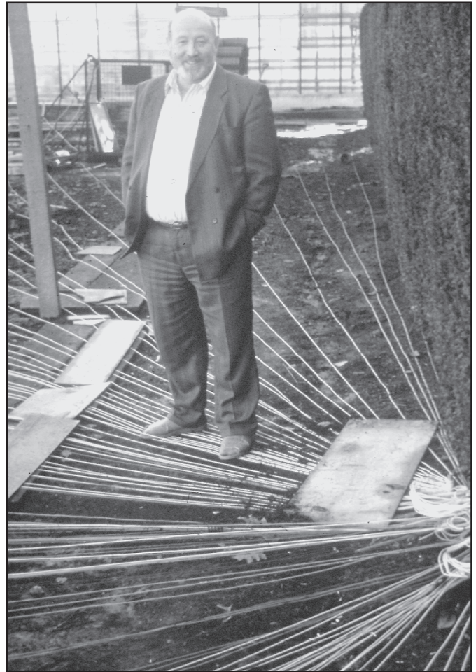
Fig 9-42—Walter Skudlarek, DJ6QT, inspecting some of the radials used on the 160-meter vertical at ON4UN. Half of the radials are buried (where the garden is), and half are just lying on the ground in the back of the garden behind the hedge (where the XYL can't see the mess from the house!). In total, some 250 radials are used, ranging in length from 15 to 75 meters.
