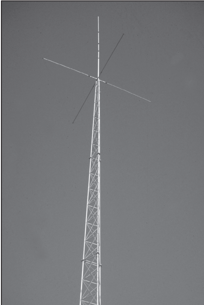
Fig 9-74 —Self-supporting 39.5-meter \lambda/4 vertical for 160 meters at ON4UN. The base is 1.8-meters wide and the tower tapers to just a few inches at the top. The tower is shunt fed with a gamma match and also serves as a support for an 80-meter Four-Square array made of \lambda/4 verticals, supported from sloping catenary lines running from the 160-meter tower.
