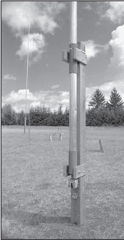
Fig 9-69—Base of one of the irrigation-pipe 80-meter verticals constructed by K7EM.
